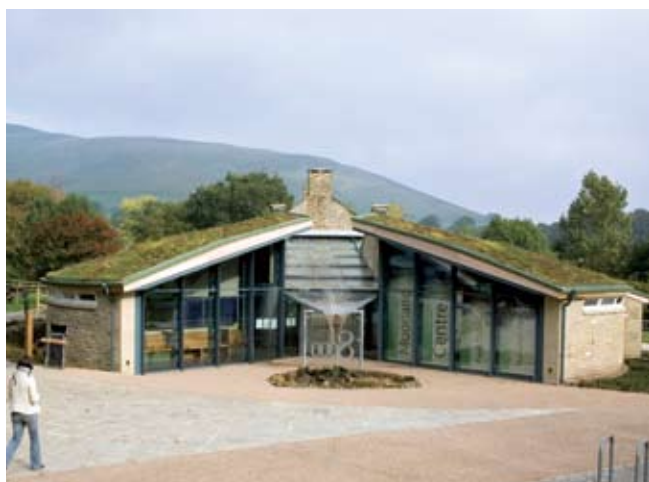
Peak District National Park's Moorland Centre reflects its upland setting. It has a living turf roof for insulation and is heated by a ground source heat pump
